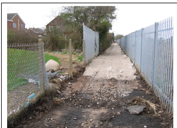
Malpas Road to Heath Road Greenway: during construction.
