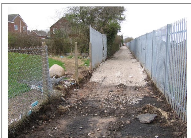
Malpas Road to Heath Road Greenway: during construction.
