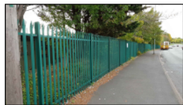
Proposed Fencing New boundary fencing to match existing along Everette Road 2.1m High Green powder-coated galvanized fencing
